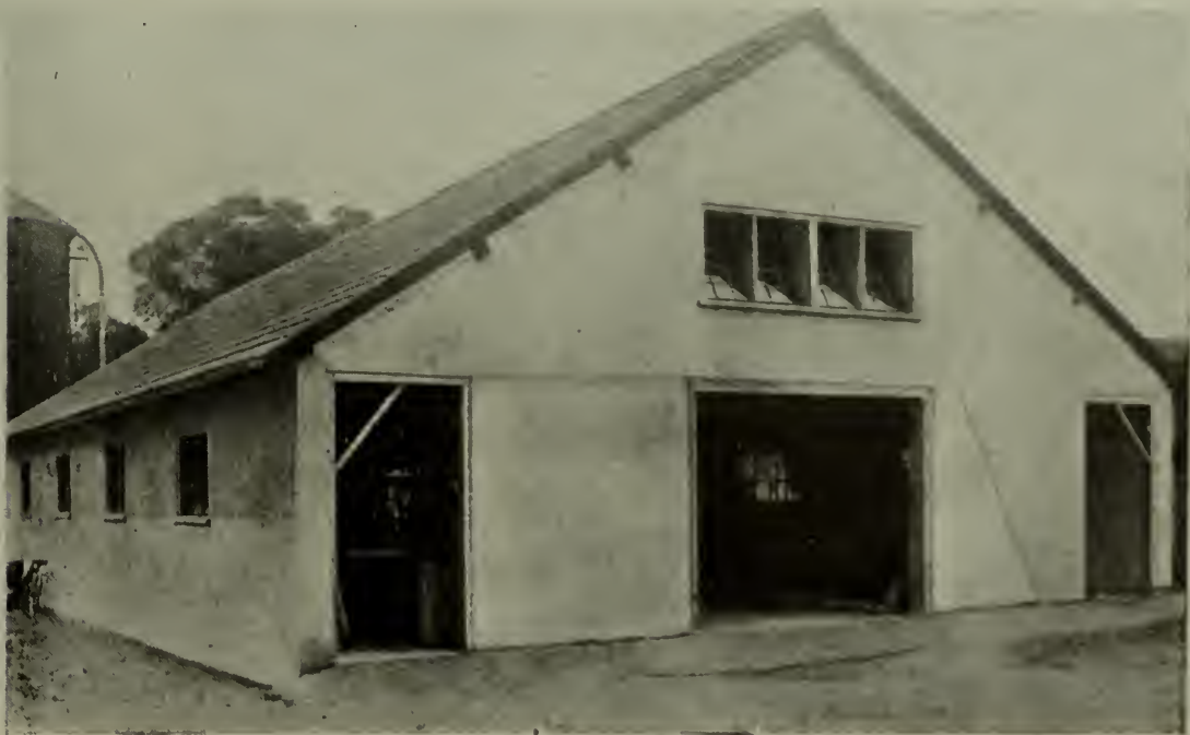
CONCRETE COW-BARN ON LORD ASTOR'S FARM, COOKHAM, BERKS.
